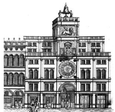
Clock Tower with the XVIII century raisings and terraces
